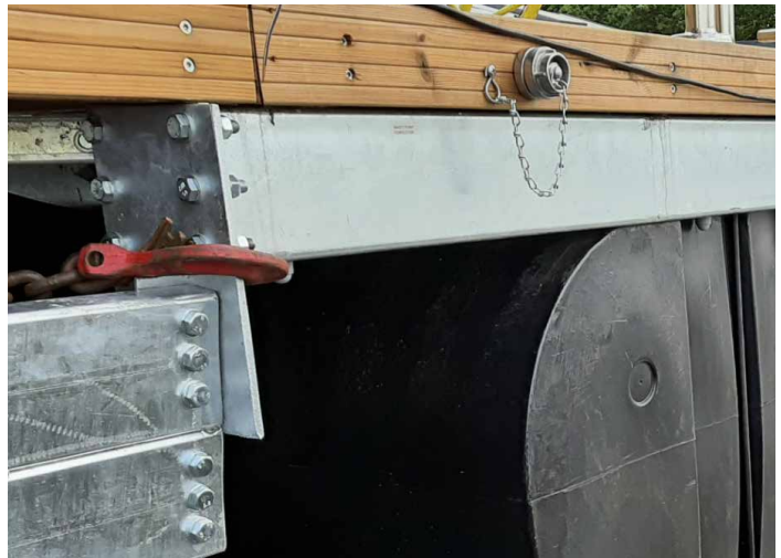
WASTE PUMP CONNECTION
